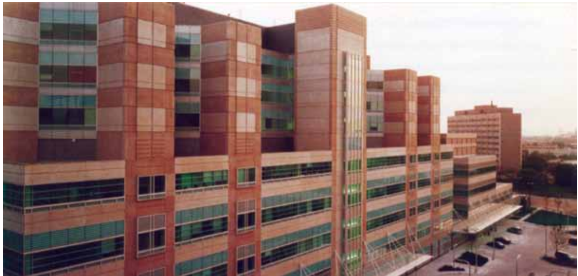
Figure 36 Insulated sandwich wall panels. John H. Stroger, Jr. Hospital of Cook County, Chicago, Ill. CCH Design Group headed by Loebel Schlossman & Hackl. (Courtesy ©Hedrick Blessing)
