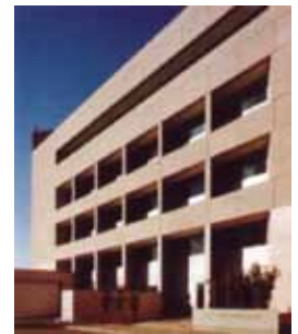
Figure 10 Deep recessed windows. (Courtesy © Glen Allison)
