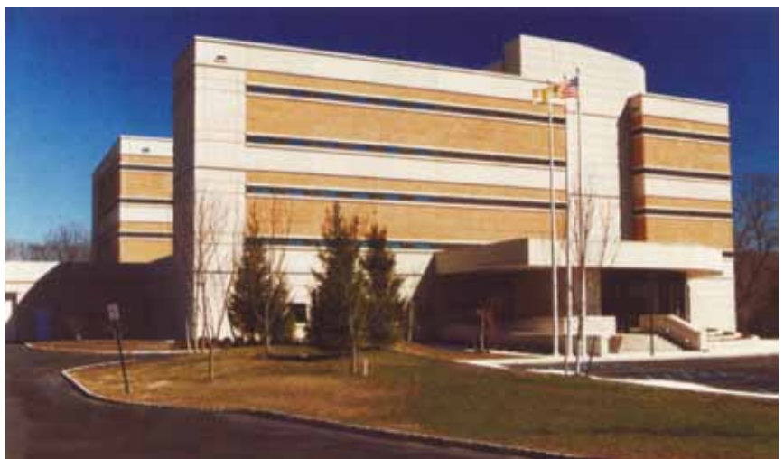
Figure 38 Insulated sandwich wall panels with exposed interior. Morris County Correctional Facility, Morris Township, NJ. Hellmuth, Obata & Kassabaum.
