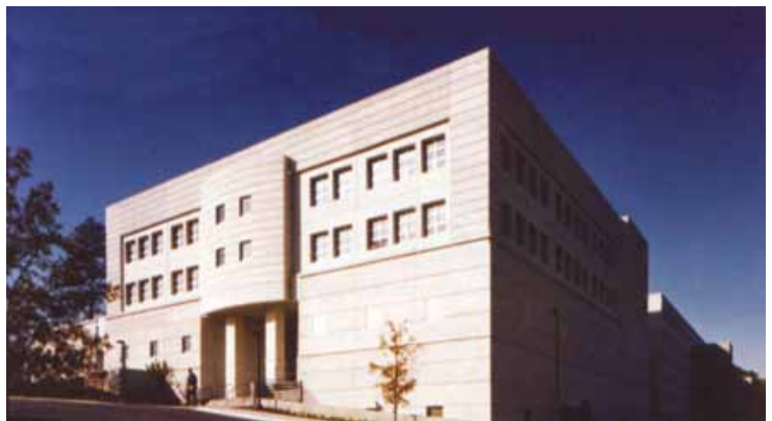
Figure 37 Insulated sandwich wall panels with exposed interior. Academic Facility for the John F. Kennedy Special Warfare Center Fort Bragg (Fayetteville), NC. LS3P Architects, Ltd.
