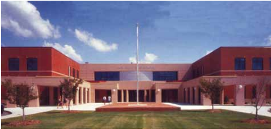
Figure 39 Insulated sandwich wall panels painted on the interior. Jack Britt High School, Fayetteville, NC. Shuller, Ferris, Lindstrom & Associates.
